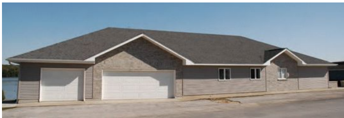
Streetside: The Harthoorn's house replaces a boarded-up garage.
